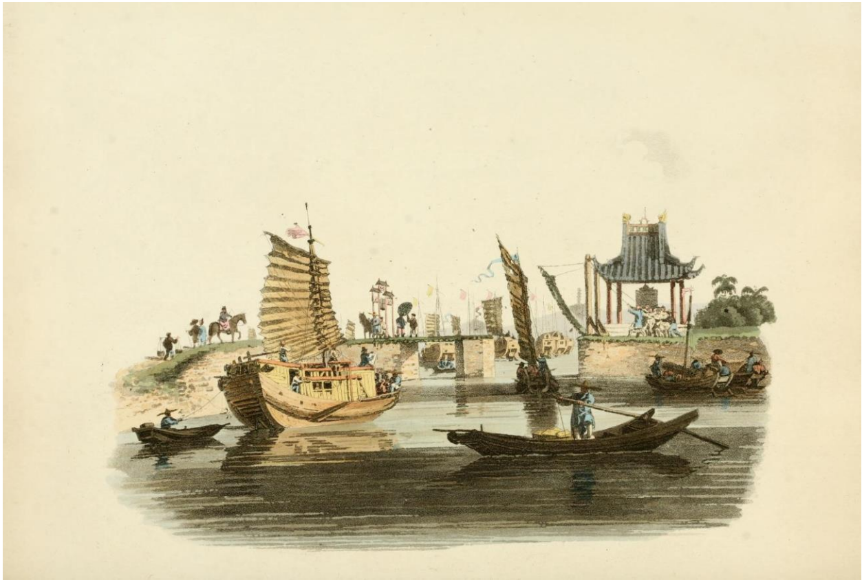
VESSELS PASSING THROUGH A SLUICE.
